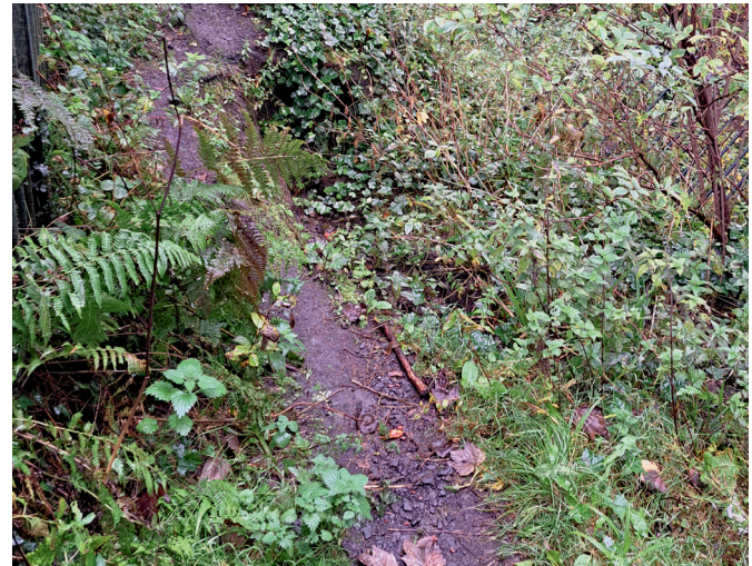
📍 Path blocked below steps with landslide beyond
